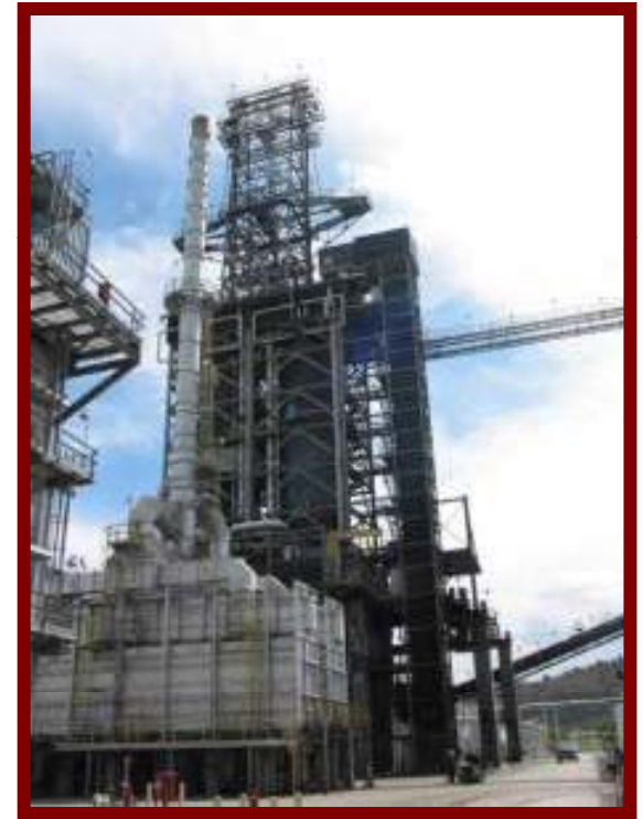
Billings Refinery Coker Courtesy of CoP
