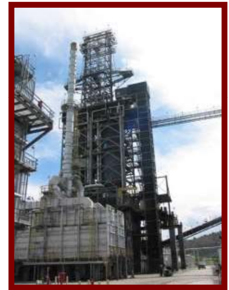
Billings Refinery Coker Courtesy of CoP
